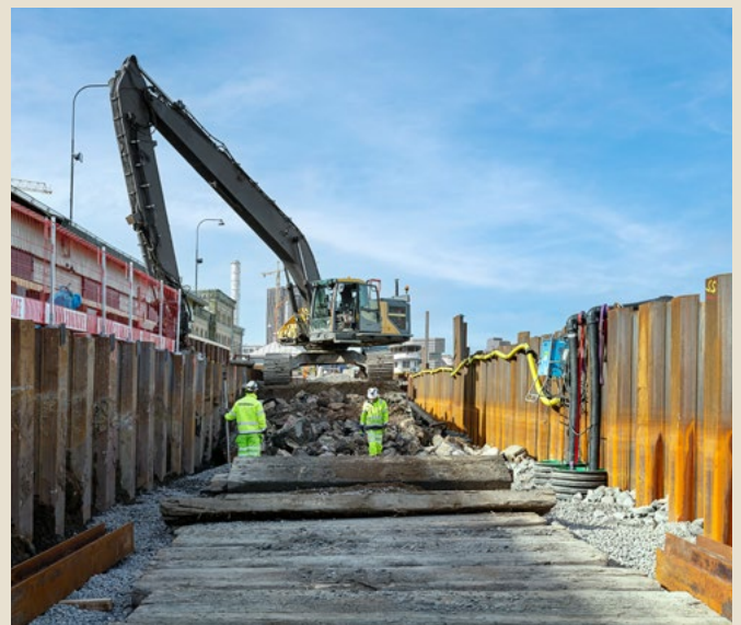
Refurbishment of Packhuskajen, measures made to withstand potential rises in sea levels.
